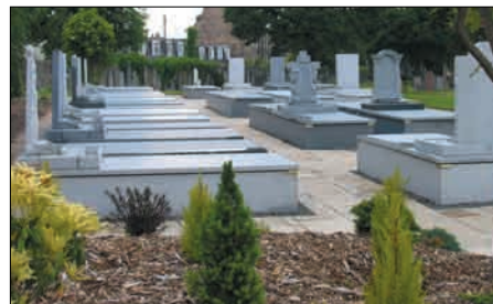
Scotland - Double Interment Chambers Partially Above Ground with Granite Cladding + Heritage Memorial Systems
