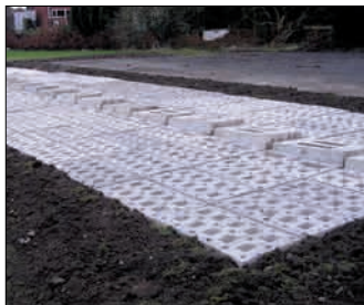
West Midlands - Double Chambers with Grass Mats and Riser Blocks
