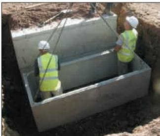
Stoke on Trent - Double Interment Ring Systems
