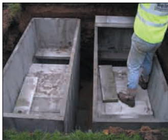
Greater Manchester - Double Interment Below Ground Burial Chambers
