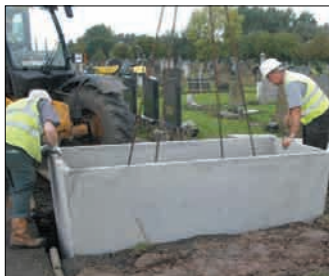
Essex - Single Interment Chamber Installation
