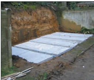
North London - Double Chambers Installed Between Existing Structures
