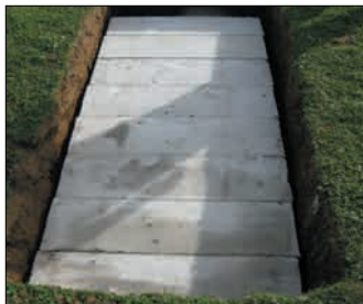
Bedfordshire - Double Interment Below Ground Chamber
