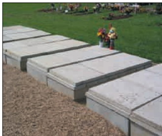
Cheshire - Double Interment Burial Chambers Partly Protruding Above Ground
