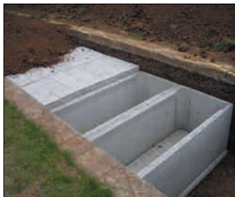
Berkshire - Interment Rings Installed on a Foundation Raft
